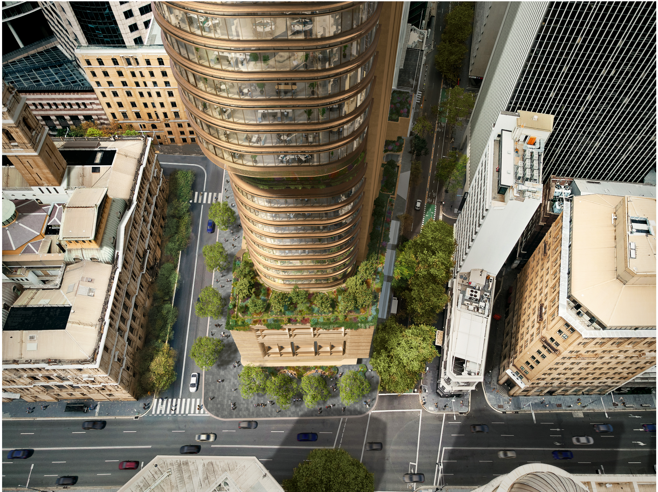
Aerial view from North
